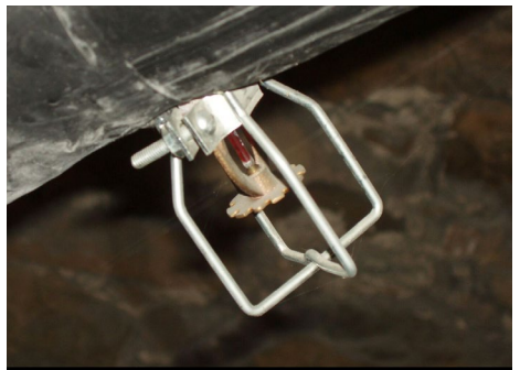
↑ As this automatic fire suppression system head is located in the attic of the A-listed Duff House it does not require to be discretely located. These heads can, however, be fully recessed with cover plates to match their backgrounds in more sensitive historic areas.
