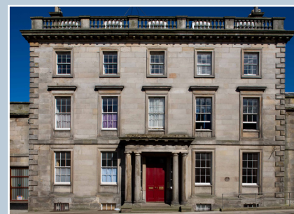
Central block of the former Fife Arms Hotel, Banff, 1843–5. The classical design places emphasis on the symmetry, proportions and detailing of the walls and reflects the functional hierarchy of the interior. Corniced windows indicate the principal rooms on the first floor; smaller windows relate to private or subsidiary rooms. The design maximises the architectural impact of the walls by hiding the shallow pitched roof behind a parapet. © N.Haynes.
