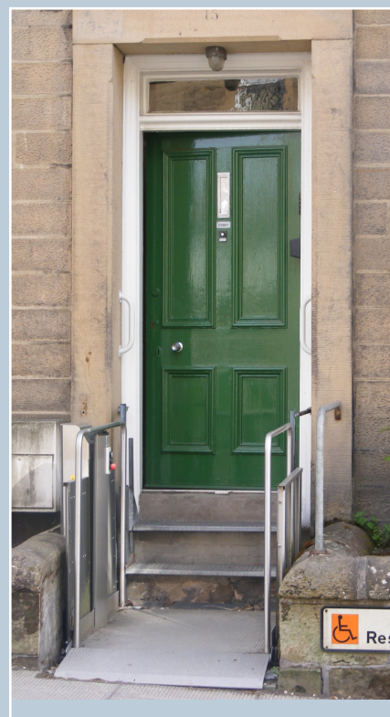
A small platform lift providing disabled access at a property in Hawick.
