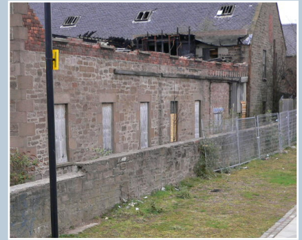
Former Arctic Tannery and Harbour Workshops, Dundee. A fire destroyed the upper part that had originally been of timber louvres to cure sealskin hides, replaced in brick. The development of housing (see below) echoes in a new form the timber and brick previously used here.
