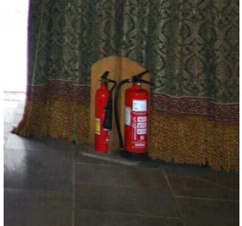
↑ Extinguisher stands in the Great Hall at Stirling Castle. By using free-standing extinguishers, any damage to the historic fabric has been minimised. © Rob Thomson
