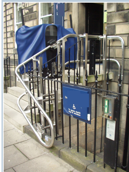
The need for user assistance, regular mechanical maintenance and obtrusive fixtures limits the suitability of external stair lifts in many locations.
