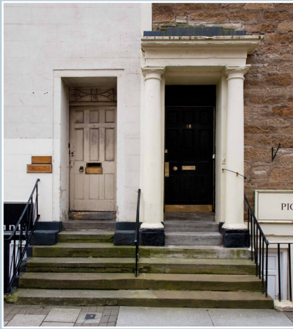
Removal of the left-hand doorcase has unbalanced this pair of entrances. © N. Haynes.
