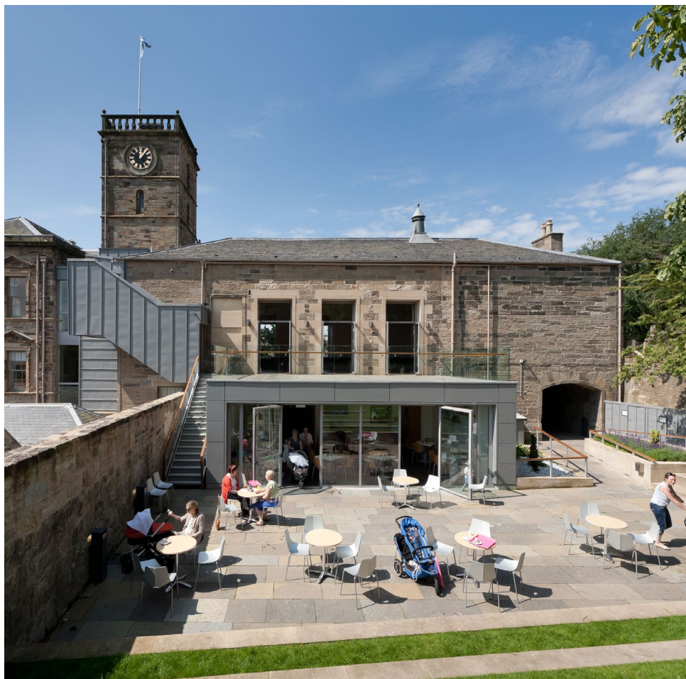
↑ Linlithgow Burgh Halls, which dates from the seventeenth century, reopened in 2011 after a substantial redevelopment. The project included a requirement to provide a new fire escape for the A-listed building. The solution here was to provide an enclosed escape stair clad in zinc. © Dave Morris Photography
