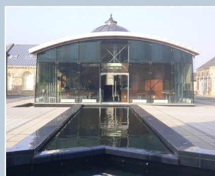
The extension to Esk Net Mills, Musselburgh, East Lothian. The glass extension of 2006 makes a deferential contrast to the solid masonry of the surrounding courtyard buildings of the 19th-century net-making complex. The design draws on the symmetry and scale of the old buildings, whilst creating a distinctive new component in its form and materials.
