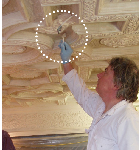
↑ An aspirating smoke-detection system was installed in the Laich Hall at Edinburgh Castle during restoration work. These systems draw air through small pipes to detect smoke. You can see the pipe here before it has been cut back to lie flush with the ceiling, forming a near-invisible detection system. © Rob Thomson
