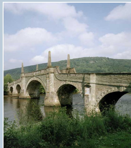
Aberfeldy Bridge, Perth & Kinross, showpiece of General Wade's military road network, combines cutwaters with neo-classical quoins and obelisks that signal the springing point of the arch. © Crown copyright: RCAHMS. Licensor www.rcahms.gov.uk .
