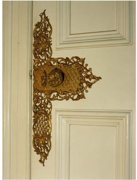
This late 19th century door handle and fingerplate at an unlisted building in Esplanade Terrace, Joppa combines beauty and practicality with its ornate design and its function in protecting the door from marks and damage. Details like this are an important part of a building's character. © Royal Commission on the Ancient and Historical Monuments of Scotland; D/12556/cn. Licensor www.scran.ac.uk
