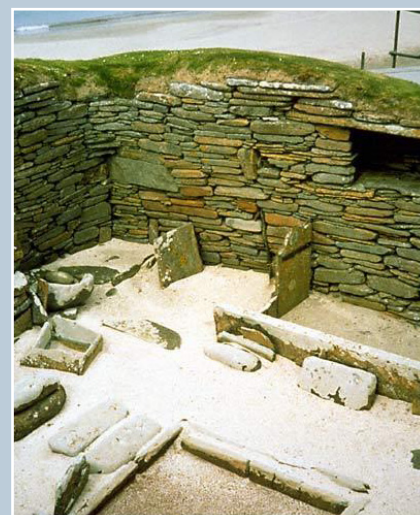
Neolithic house, Skara Brae, Orkney. From the earliest times walls were designed to provide shelter and security, to contain warmth, and to meet the functional requirements of domestic and ritual life. Local materials and skill traditions established different patterns of wall construction and building design in different parts of the country, and adapted to new types of building and usage over time.
